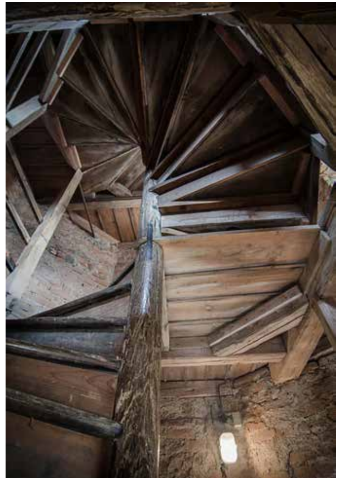
Castle Grondo: this somewhat irregular wooden spiral staircase leads to the lookout on the highest tower. Photo Mike Scott
